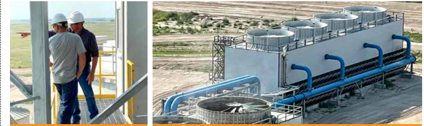
LEFT: Mitch Feldman, KAAPA Ethanol Ravenna Plant Manager, (right) discusses the facility with Dawson PPD Lineman Jerry Folck from the top of its largest grain bin. RIGHT: KAAPA Ethanol Ravenna replaced its chillers with this new cooling tower in 2021. By making this investment, the facility is estimated to reduce its electrical energy use by 1 million kilowatt-hours annually.
