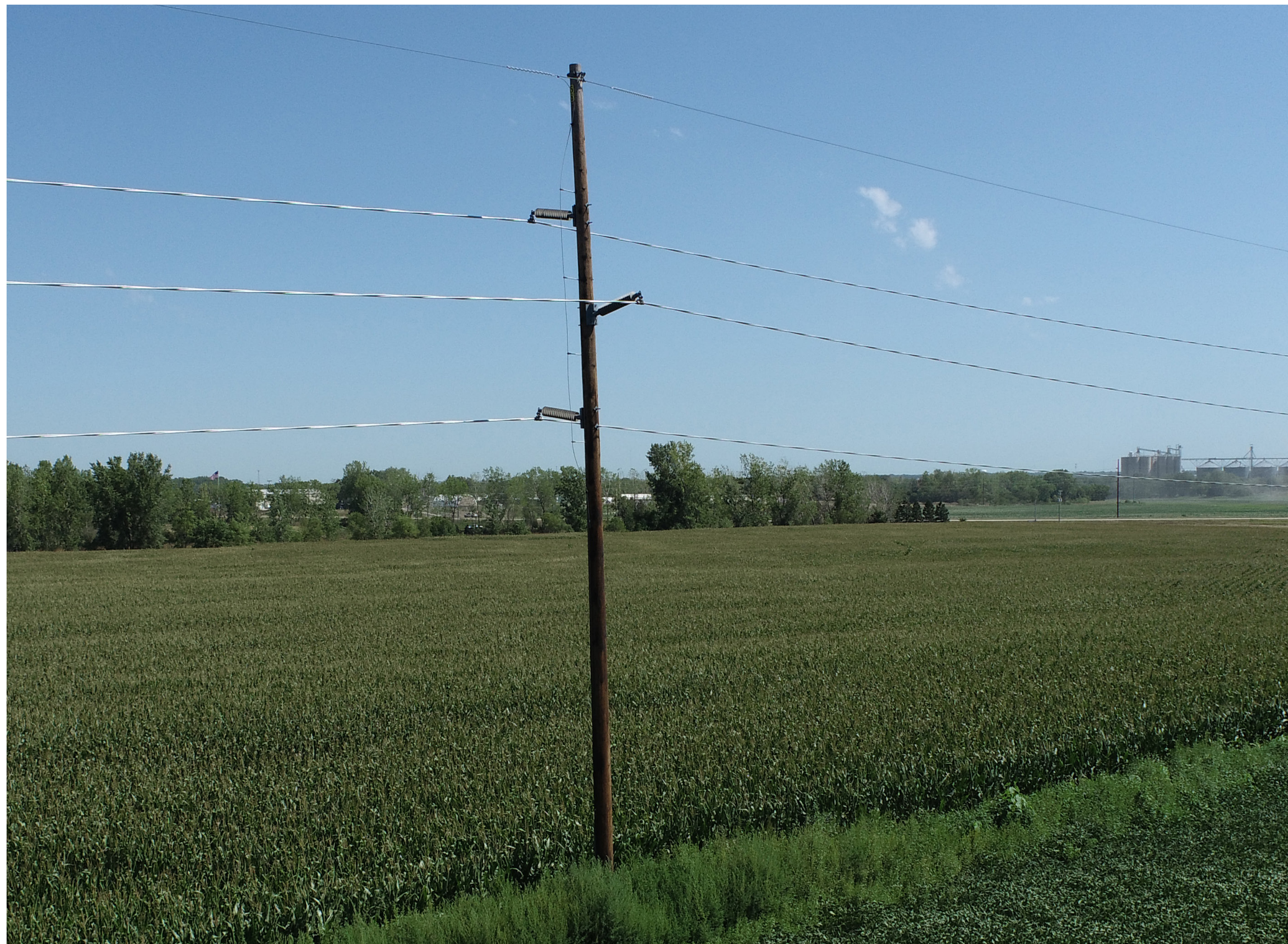
TYPICAL SINGLE-POLE WOOD STRUCTURE
