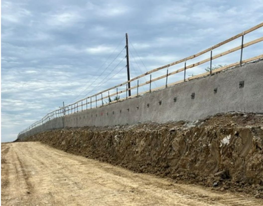
Nail Wall Construction – just south of Princeton Rd
