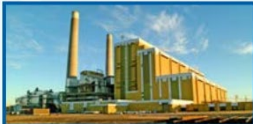
Evaluate Carbon Capture at Gerald Gentleman Station (GGS) Unit 2.
