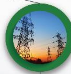
Transmission and Distribution Infrastructure
