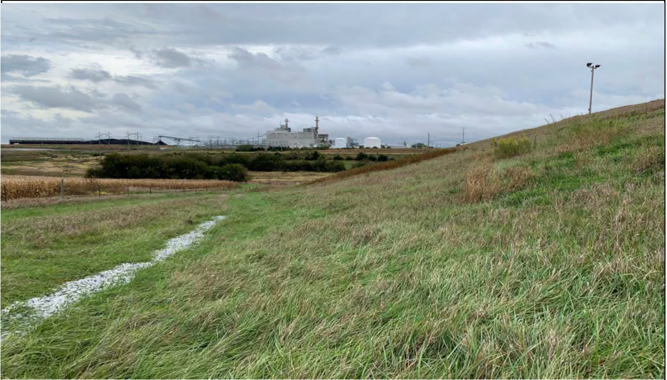
Photograph 8 Vegetation on northern exterior slope with riprap in high traffic areas. (IMG_2019.JPG)
