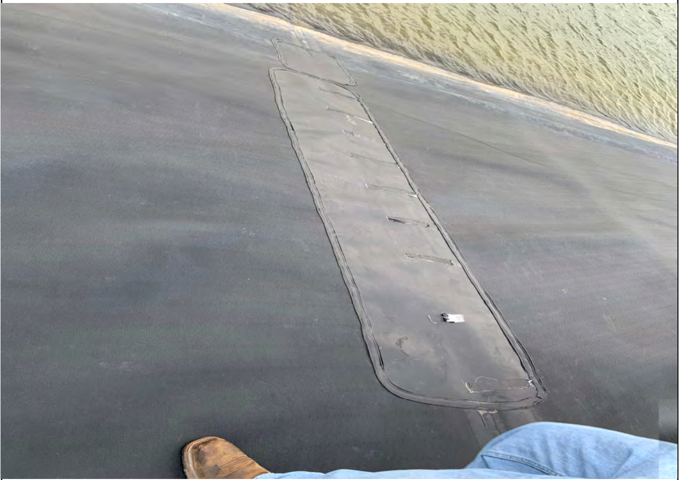
Photograph 11 Liner repair performed on leachate evaporation pond in 2019. (IMG_2034.JPG)
