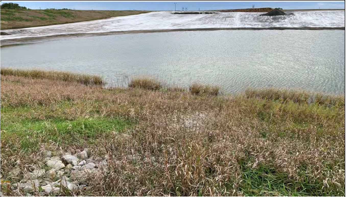
Photograph 3 Emergency overflow riprap from leachate evaporation pond to ash disposal facility. (IMG_1996.JPG)
