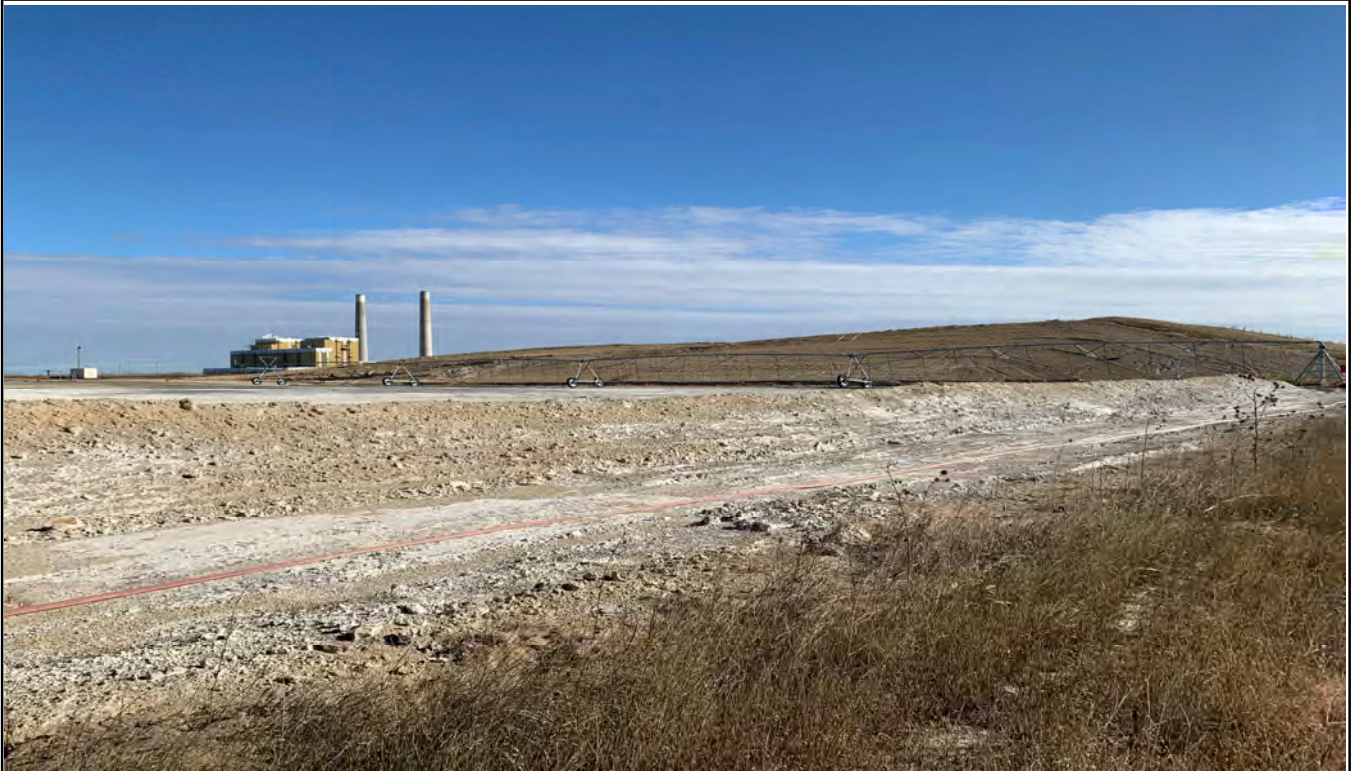
Photograph 9 Active fly ash deposition area with dust control equipment in Ash Landfill No. 3. (IMG_2119.JPG)
