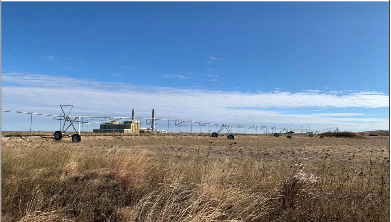
Photograph 6 Dust control center pivot at Ash Landfill No. 3. (IMG_2103.JPG)
