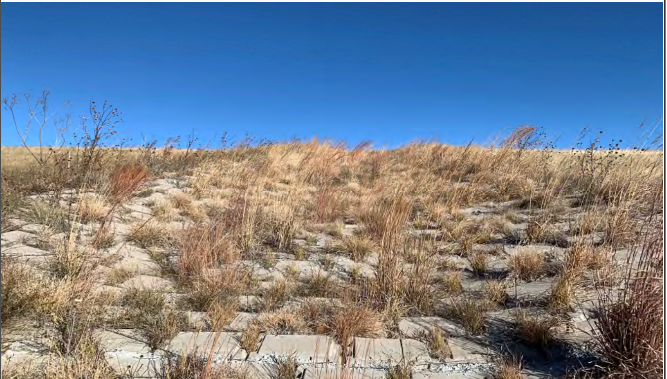
Photograph 12 Downchute channel on south side of Ash Landfill No. 4. (IMG_2128.JPG)
